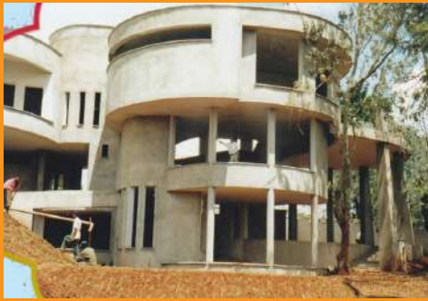
Year : 2007 | Client : Mr. Asif Padamshi Project : Construction Of 1 No Bungalow Location: At Nyari Estate Architects : Studio Infinity Architects Engineers : Eng. Simon Njoroge Gichuhi Contract Sum : 4,462,950 | Contract Period : 38 Weeks
