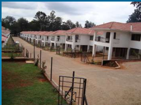
Year : 2007 | Client : Jambo Holding Ltd Project : Construction of 22 No Maisonnets Location Of Project : Grevillea Grove, Westlands Architects : Fnda Architects Inc (K) Engineers : Steel Graphics Associates Contract Sum : 162,700,000
