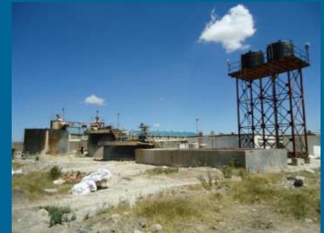
Year: 2009 | Client : Kapa Oil Refineries Ltd Project : Construction Of Sewer Line and Pump House Project: Along Mombasa Rd, Nairobi Architects: Jap International Ltd Engineers: Midrock Consulting Engineers Contract Sum : 34,949,593.00
