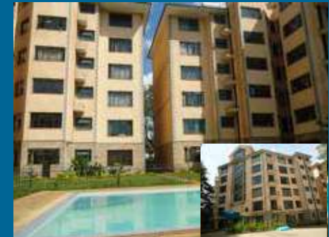
Year : 2014 | Client : Acta Holdings Ltd Project : New Construction of 24 No Luxurious Flats Location: Elgeyo Marakwet Road (Kilimani) | Architects : Wachoraji Associates Engineers : Metrix Consultants Ltd Contract Sum : 164,501,454 | Contract Period : 52 Weeks
