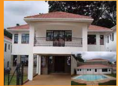
Year : 2007 | Client : Jambo Holdings Project : New Construction of 22 No Maisonettes Location: Greivillia Grove Westlands, Nairobi (Greivillia Grove 2) Architects : FNDA Architects Inc Engineers : Steel Graphics Associates Contract Sum : 162,700,000 | Contract Period : 42 Weeks
