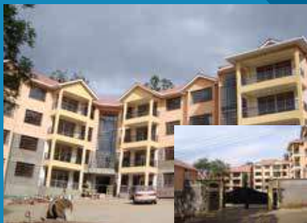
Year : 2008 | Client : Amber Investments Ltd Project : New Construction of 34 No Luxurious Residential Apartments | Location: O° R iara Road 1, Nairobi Architects : Archgrid Systems Engineers : Pharma Consulting Engineers Contract Sum : 114,118,740 | Contract Period : 48 Weeks
