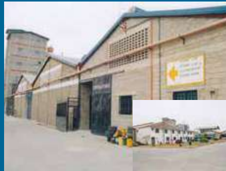
Client: Kapa Oil Project: Kapa Oil Refineries Location: Syokimau
