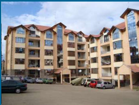
Year : 2007 | Client : Oloitoktok Ltd Project : Construction Of 17 No Luxurious Apartments | Location: O° Oloitoktok Road Architects : Archscapes Consultants Engineers : Lemager & Partners Engineers Contract Sum : 91,500,000.00
