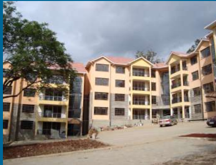
Year : 2008 | Client : Amber Investments Ltd Nature Of Project: Construction Of 34 Luxurious Apartments Location Of Project : O° R iara Road, Nairobi Architects : Archgrid Systems Engineers : Pharma Consulting Engineering Contract Sum : 148,118,740.00
