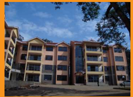
Year : 2011 | Client : Amber Properties Ltd Project : Construction Of 25 No. Luxurious Residential Apartments | Location: O° R iara Close Architects : Archgrid Systems Engineers : Pharma Consulting Engineers
