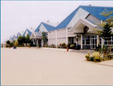
Year : 2001 | Client : E.P.Z – Capital Industrial Park Project : New Construction of 9 Go-downs Location of Project : Athi-river Architects : Design Team Architects Engineers : Pace Associates
