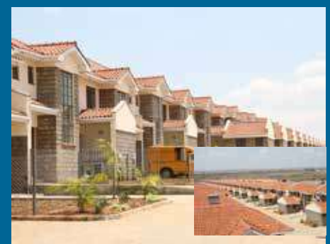
Year : 2012 | Client : Delta Corp E.A Ltd Project : New Construction of 153 Nos Luxurious Town Houses and Shopping Mall | Location: Mlolongo (Athiriver), Mombasa Road Architects : Innovative Planning & Design Consultants Engineers : Wandua Consultants Contract Sum : 623,450,847 | Contract Period : 74 Weeks
