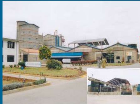
Year : 2011 | Client : Kapa Oil Refineries Ltd Project : Construction Of New Godowns & New Soap Plant Project : O' M ombasa Road | Architects : Jap International Ltd Engineers : Midrock Consulting Engineers Contract Sum : 29,117,076.50
