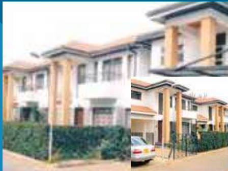
Year : 2006 | Client : Jambo Holdings Ltd | Project : Construction of 10 No Maisonnets Location: Brookside Drive, Brookside Architects : Fnda Architects Inc (K) Engineers : Steel Graphics Associates Contract Sum : 71,200,000.00
