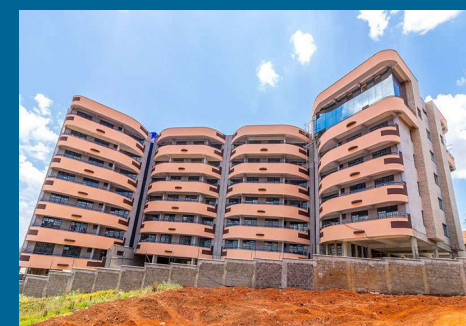
Year : 2017 | Client : Krishna Sky 09 Ltd Project : 72 Residential Apartments Location Of Project : Kabarsiran Avenue, Lavington Architects : Tana & Associates Ltd | Engineers : Pleng (K) Ltd Contract Sum : 526,276,810.00 Contract Period : 78 Weeks
