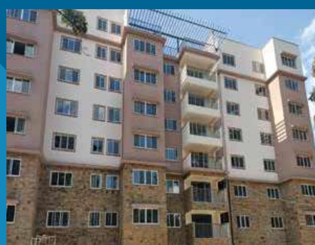
Project : Gitanga Road Apartments
