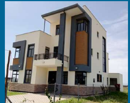
Location: Syokimau House
