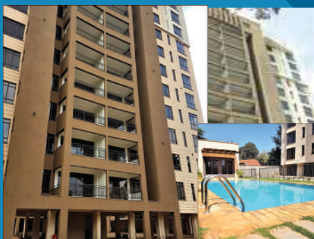
Year : 2017 | Client : Amber Properties Ltd Project : 48 Residential Apartments Location Of Project : Othaya Road, Lavington Architects : Studio Injnyity Architects Contract Sum : 480,724,999.00 | Contract Period : 76 Weeks
