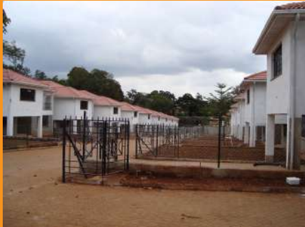
Year : 2008 | Client : Jambo Holdings Ltd Nature Of Project : Construction of 15 No Maisonettes Location: Greivillia Grove, Brookside Architects : Fnda Architects Inc (K) Engineers : Steel Graphics Associates Contract Sum : 110,615,000.00
